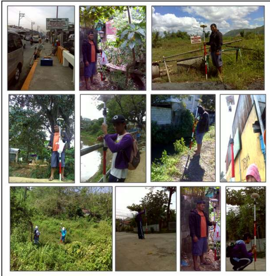
Figure 46. Pictures showing the conduct of profile and cross-section surveys in Ampid River which is a tributary of Marikina River.
