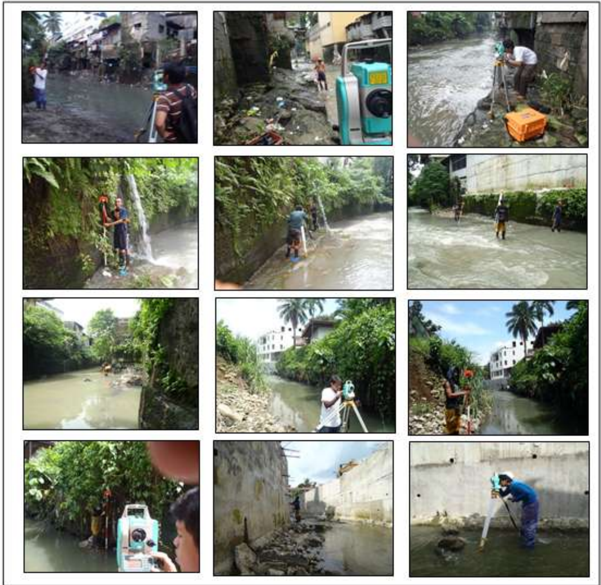
Figure 49. Pictures showing the conduct of profile and cross-section surveys in Mariblo Creek which is a tributary of San Juan River.
